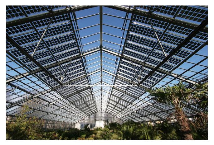
Preventing overheating in glass houses by partially shading PV modules
